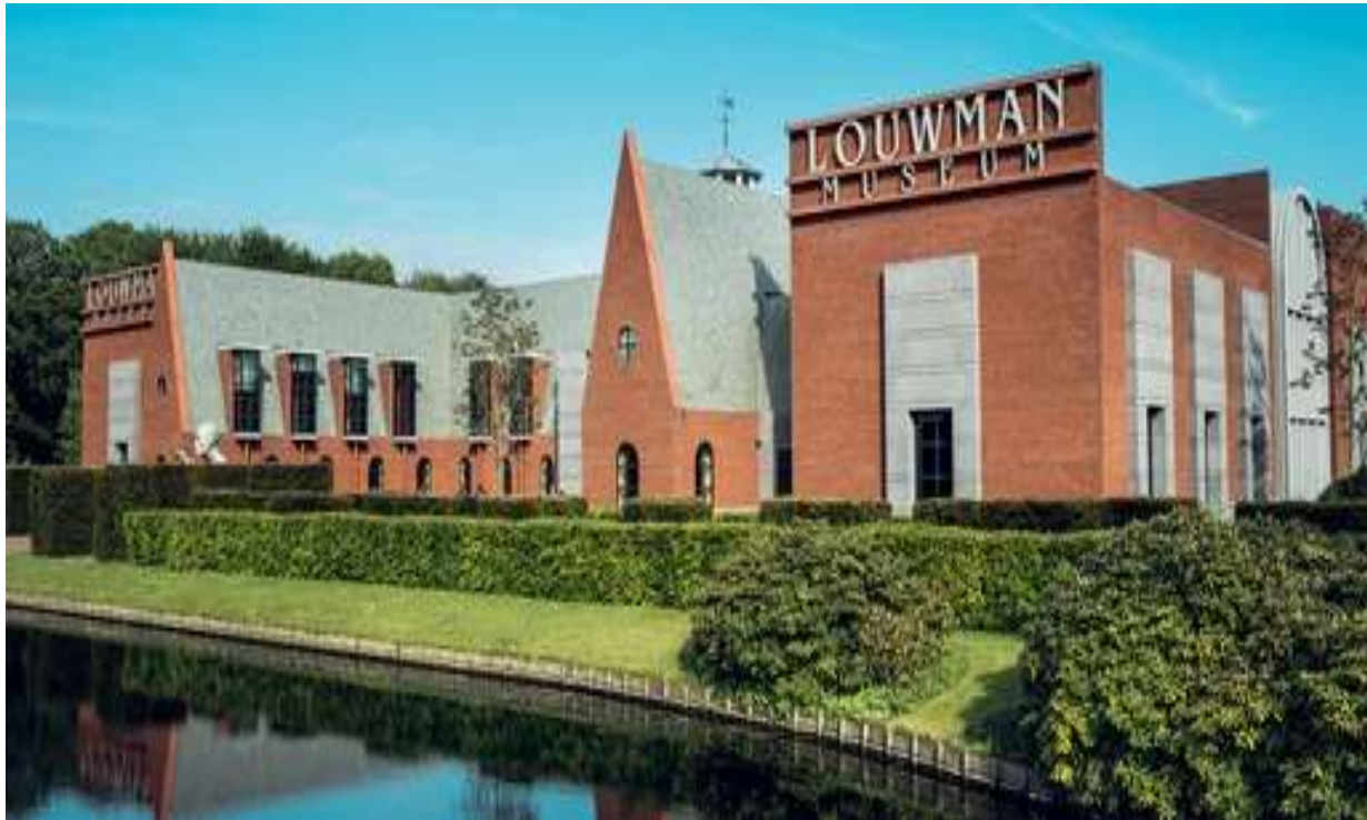
Figure 5.1 The unique architectural building design of the Louwman Museum
