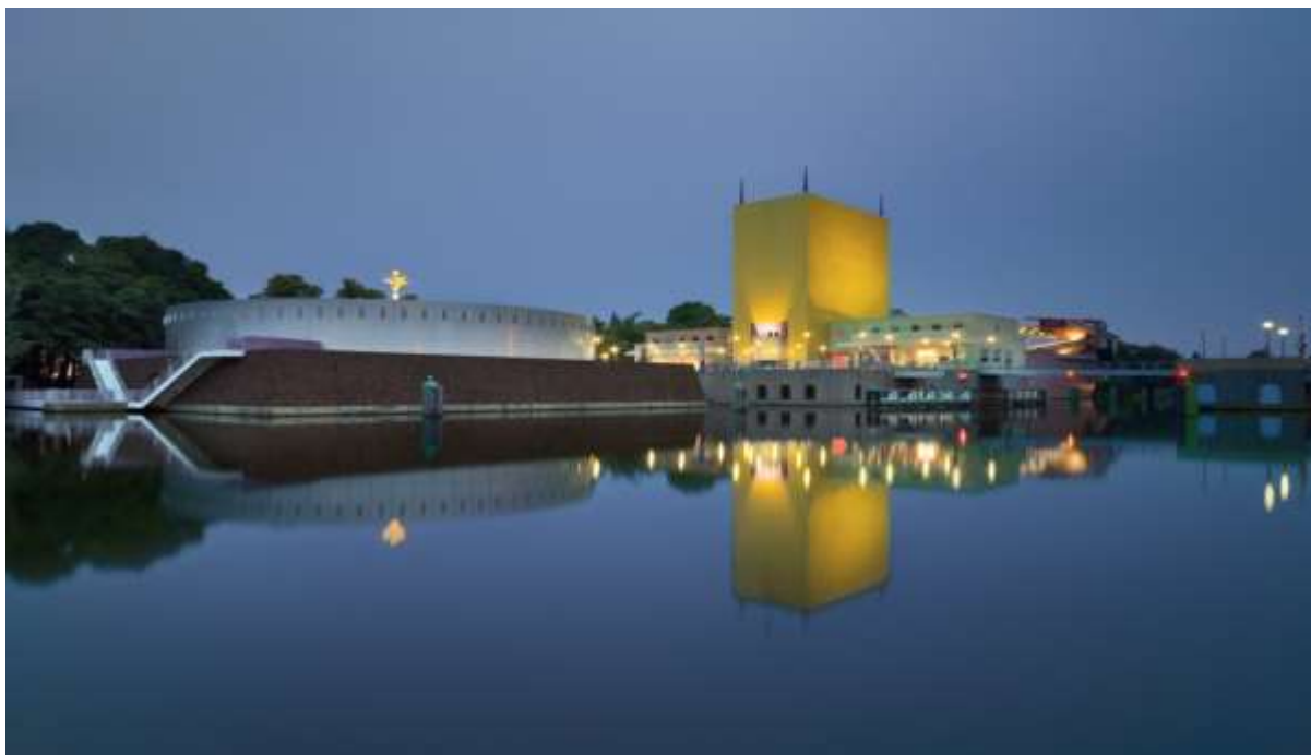
Figure 5.6 Groninger Museum astounding night building view
