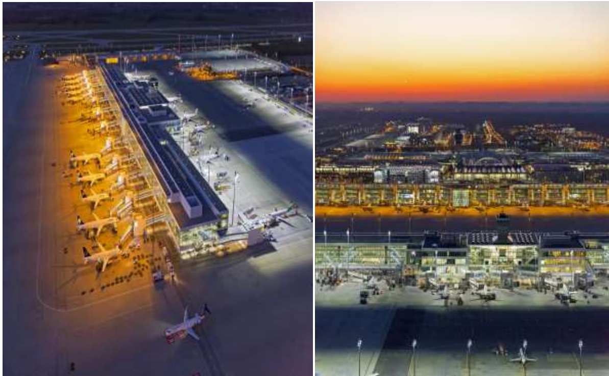
Figure 6.9 Munich Airport’s state-of-the-art aircraft arrival terminals infrastructure
