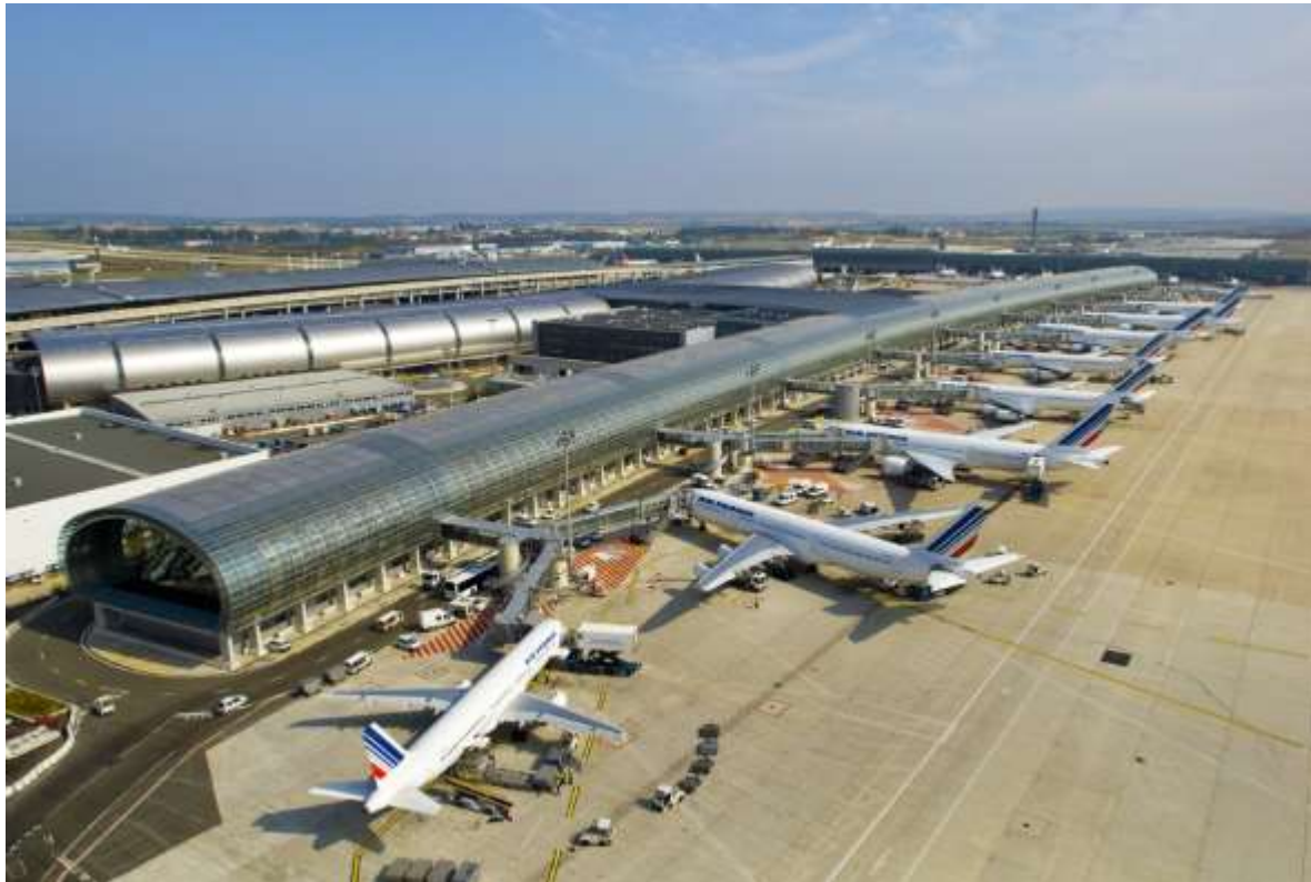
Figure 6.2 Paris-Charles de Gaulle Airport astounding world class climate friendly infrastructure facilities
